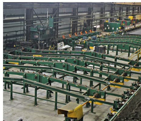
Drag Chain Skid for Pipe Cooling Bed
