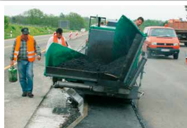
SURFACING MEDIAN STRIPS ON MOTORWAYS
