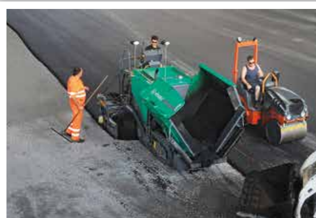
PAVING WORK IN SPORTS FACILITIES
