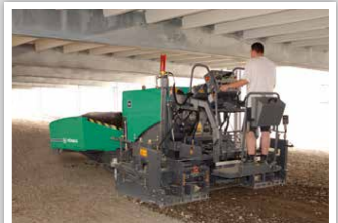
BUILDING THE BASE FOR PAVING SETTS
