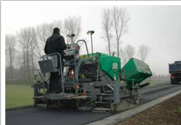
PAVING ASPHALT ON DAMS
