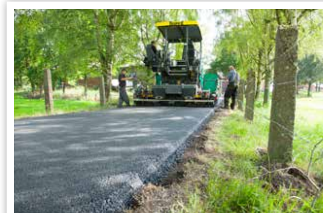
PAVEMENT REHABILITATION ON ACCESS ROADS
