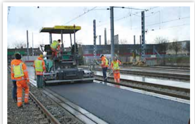
ASPHALT PAVING ON RAILWAY PLATFORMS
