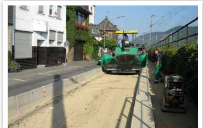
PAVEMENT REHABILITATION ON MUNICIPAL ROADS
